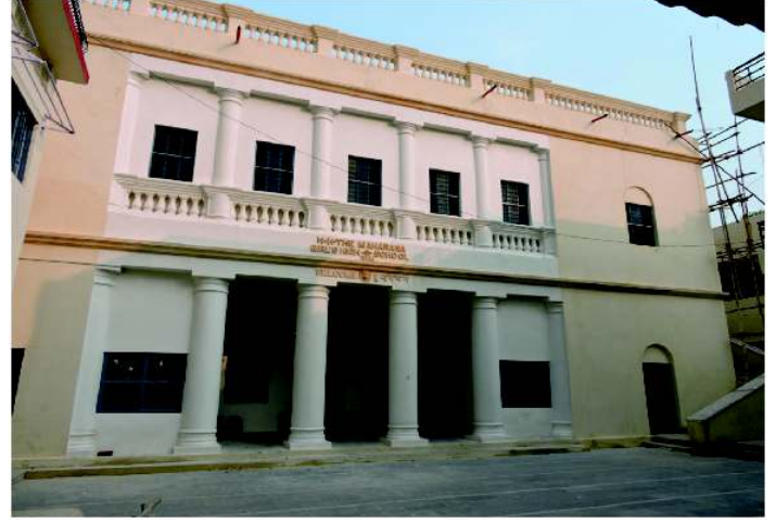
After (Western Facade)
