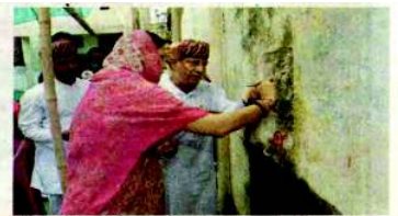
Nivritti Kumari Mewar of Udaipur is seen starting the restoration work of the school building
