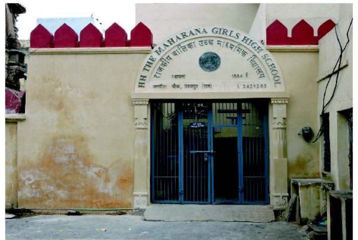
After (Main Entrance)
