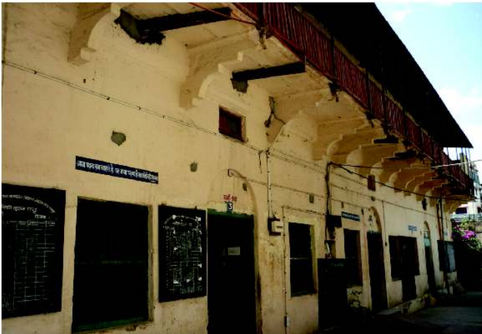
Before (Eastern Facade)
