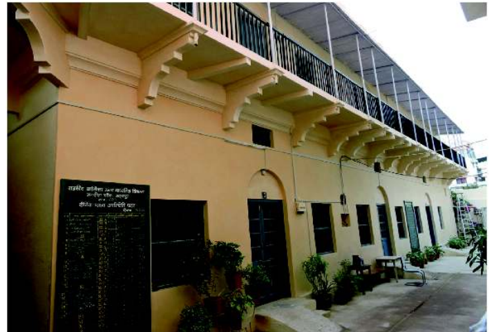
After (Eastern Facade)
