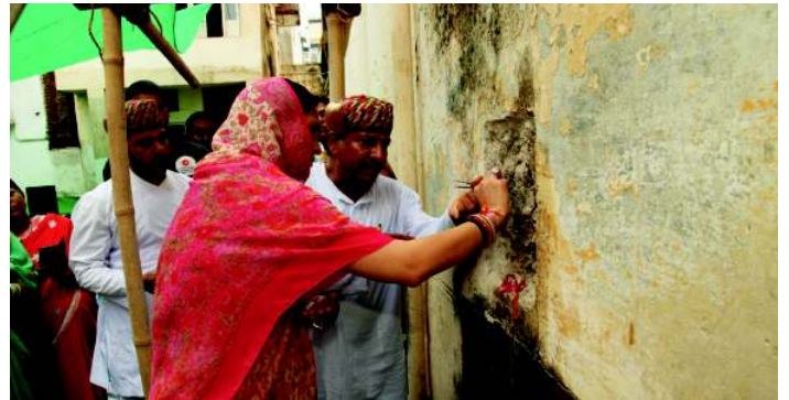
Ms. Nivritti Kumari Mewar of Udaipur is seen starting the restoration work of school building by putting lime on the wall on 17th July 2014 as per the mahurat at 11.30 am
